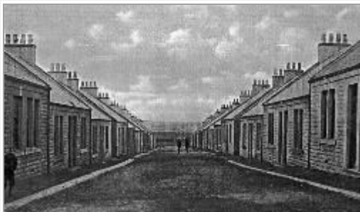
Waverley St, Lochore. Built 1909 by Fife Coal Co Ltd. 16 houses of 3 apartments and 32 houses of 2 apartments with sculleries & WC. [1926 description]
