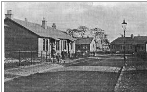
Montrose Cres, Lochore. Built by Fife Coal Co Ltd in 1924 to 1925. 102 houses with 3 rooms, bathroom, WC, hot and cold water, larder and scullery with copper. [1926 description]
